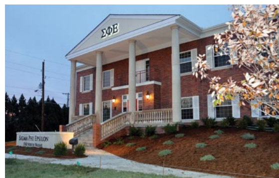
Wichita State's newly built facility will house 32 men. Above, the chapter library offers an impressive space for meetings and studying. The balcony holds numerous tables and chairs for small study groups.
